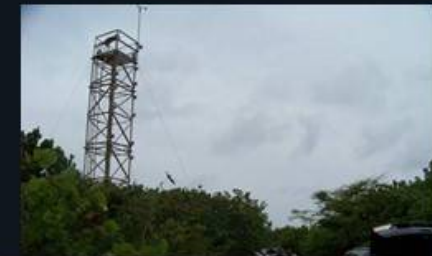
Sandy Point Weather Station, St. Croix, damaged but not silent
