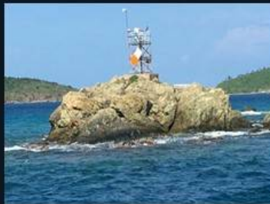
Two Brothers Weather Station, St. John, damaged and silent
